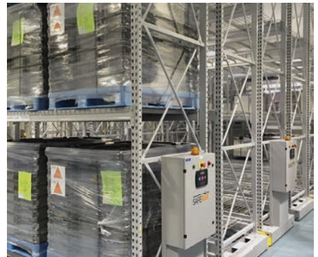
SAFERAK® 32P POWERED MOBILE RACKING SYSTEM FOR COLD STORAGE Sanofi Pasteur, Swiftwater, PA
